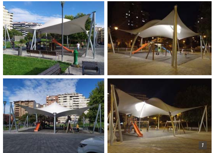
Figure 1. The tensile cover for the playground in Azpilagaña
