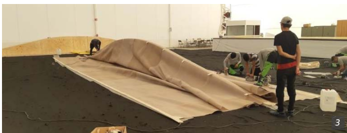
Figure 3. Fabrication process showing two sections of fabric being connected to the wooden frame.
