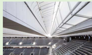
Retractable roof Philippe Chatrier © DVVD Architectes
