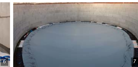
Figure 1. The aerial view of the biogas plant Figure 2. The floating deck under construction Figure 3. Detail of the steel reinforcement Figure 4. The positioning of the membrane roof Figure 5. The membrane roof ready to be deployed Figure 6. The detail of the tensioning system and the protective layers around the perimeter of the floating deck Figure 7. The tensioned membrane roof
